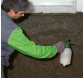
Priming with KÖSTER Polysil TG 500
