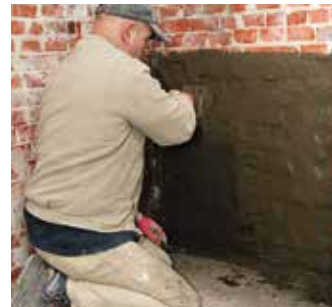
4 KÖSTER KD 1 Base: in 2 coats (second layer after 30 minutes)
