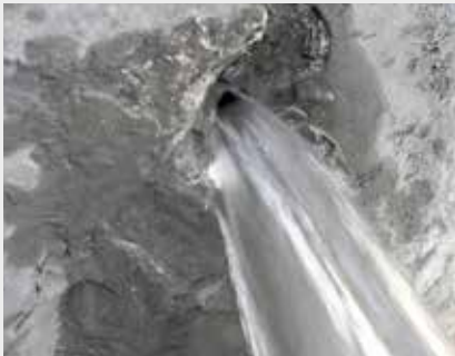
An active leakage is sealed instantly after applying KÖSTER KD 2 Blitz Powder.
