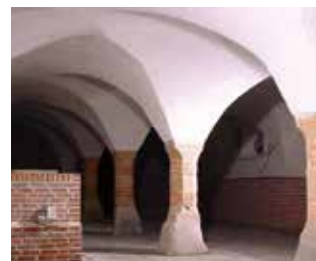
The interior walls of these buildings were restored with KÖSTER Restoration Plaster White.
