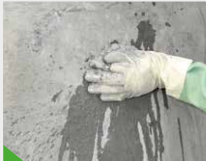
An active leakage is sealed instantly after applying KÖSTER KD 2 Blitz Powder.
